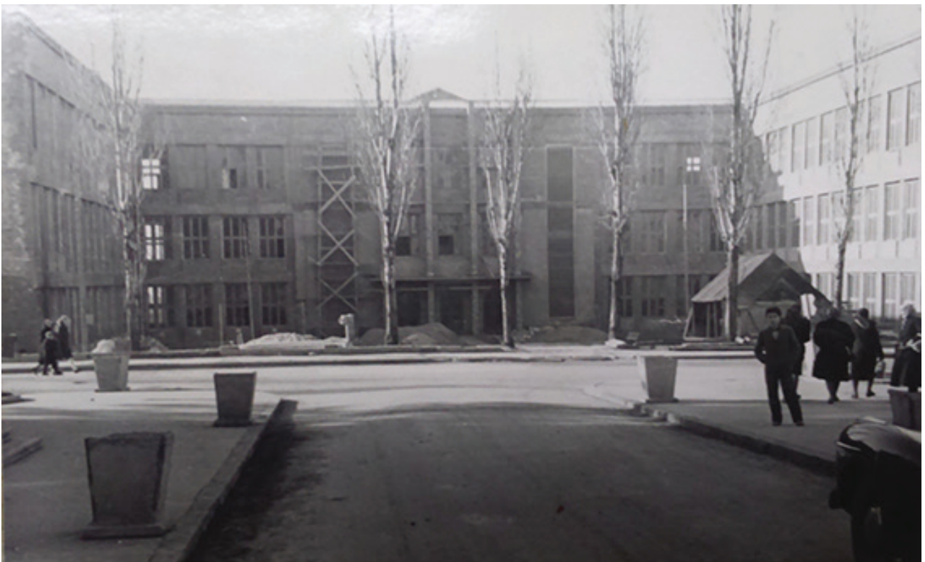
Figure 2. Construction and reconstruction of the building of the Institute of Physiology and Histology (Archives of Yugoslavia, Committee for the Protection of Public Health / Φ-31 / United Yugoslav Relief Fund of America, Extracts from Field Trip Report of Phillip E. Nelbach, Executive Director, May 13, 1948)
